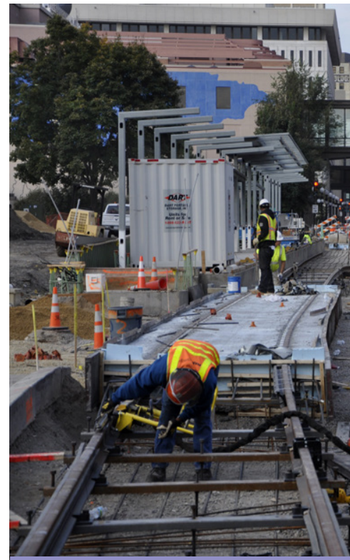
Construction during the Green Line project, Minneapolis, MN
